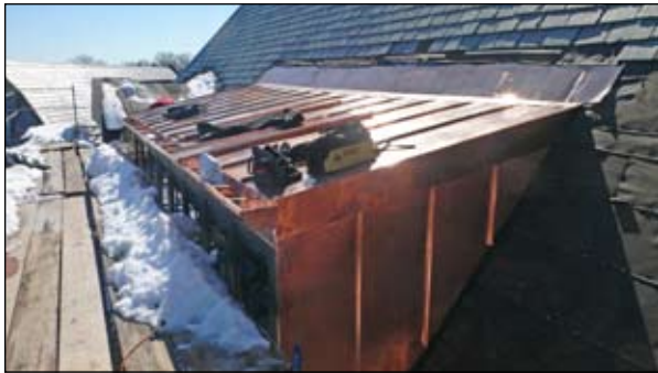
Shed Roof Replacement - Under Construction
